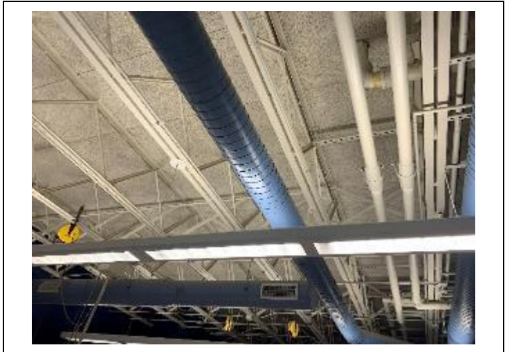
16. Tectum roof deck. No asbestos detected.
