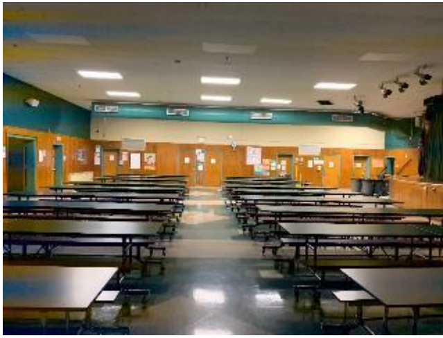
7. Cafeteria with 12" floor tile and ACBM black flooring mastic.
