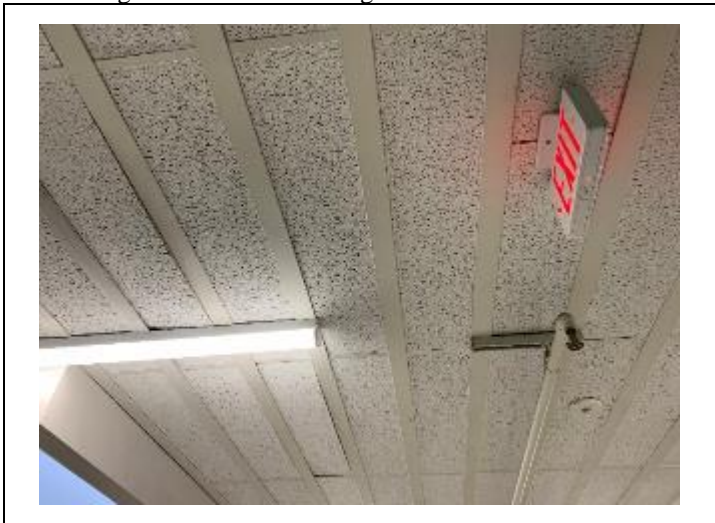
17. Suspended ceiling tiles throughout. No asbestos detected.
