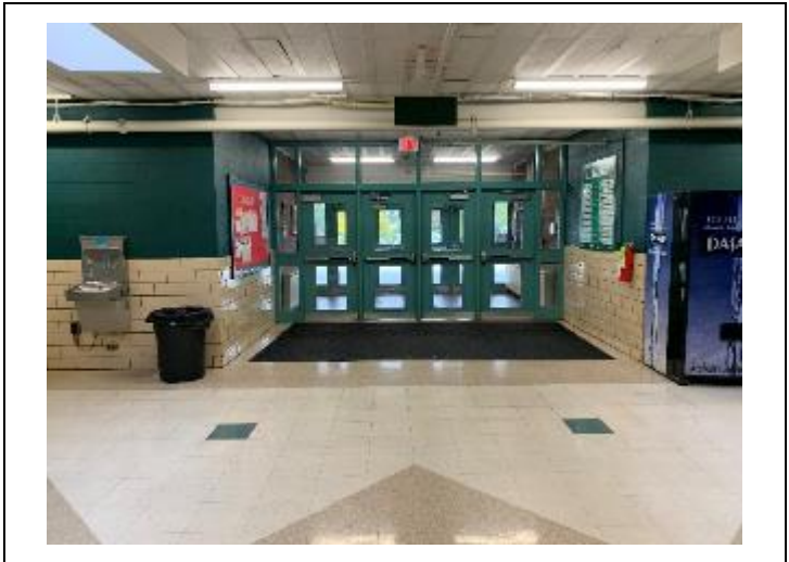
6. Entrance with 12" floor tile with ACBM black flooring mastic.
