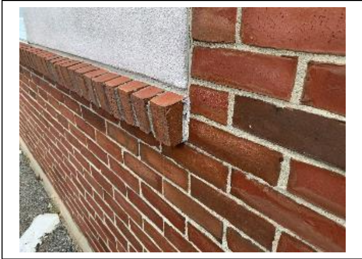
3. Exterior window caulk. No asbestos detected.
