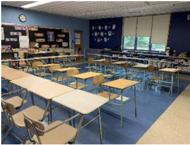
9. Classroom with ACBM flooring mastic and ACBM chalkboard with assumed ACBM glue daubs.
