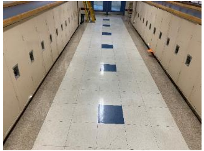
10. Hallway with 12" floor tile and ACBM black flooring mastic.
