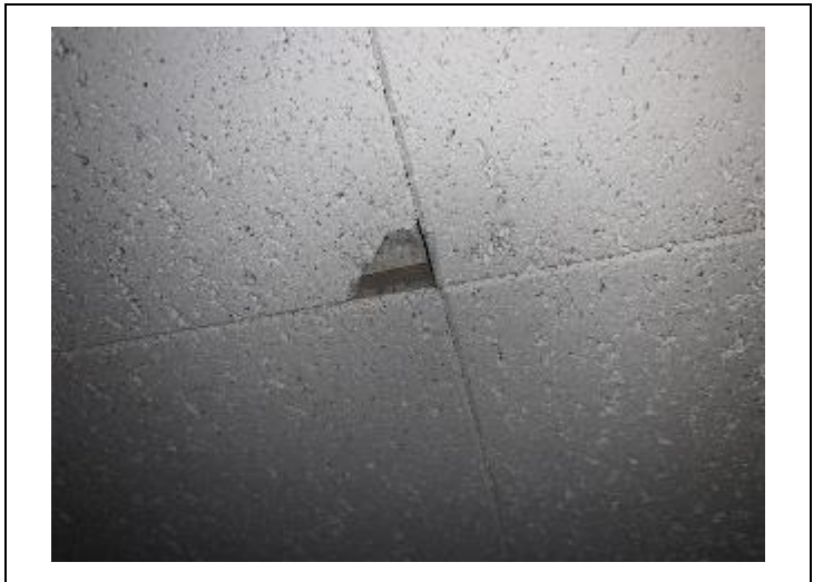
18. 12" fixed ceiling tile within room 105 storage room. No asbestos detected.
